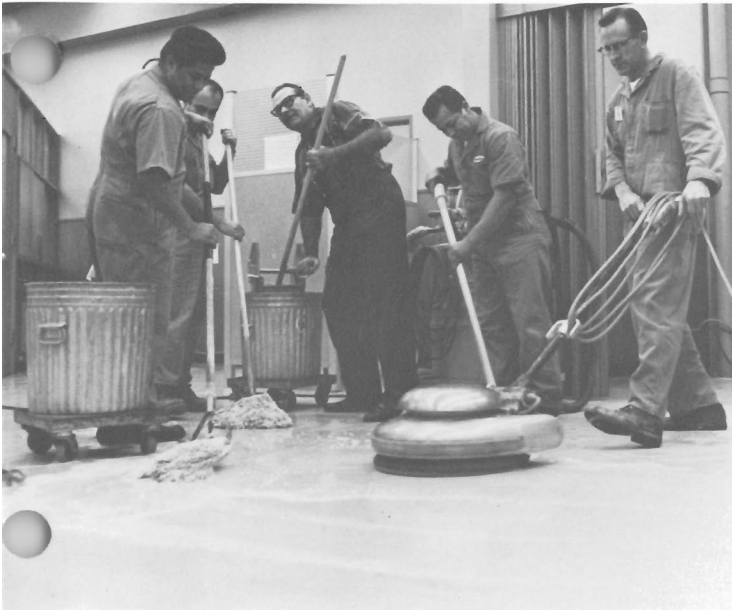
After this complete refinishing job, floors can go for years without major attention, thanks to daily cleaning and polishing. From left are Ernie Gonzales, Bart Castorena, Howard Sharboneau, Tony Mendoza, and Cal England.
